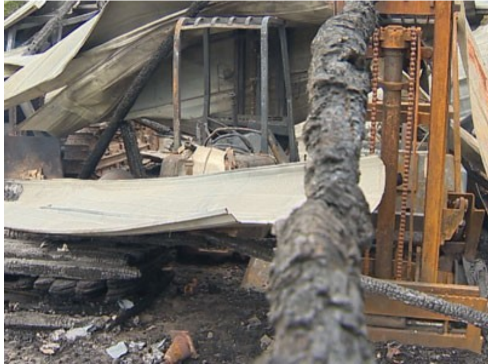
Arson is now suspected in the conflagration that destroyed buildings and vehicles in a fire in storage yard. A witness reports a number of people, believed to be migrant workers, were seen in the yard on Thursday night, the night that the fire began. The fire continued to burn through Friday.
