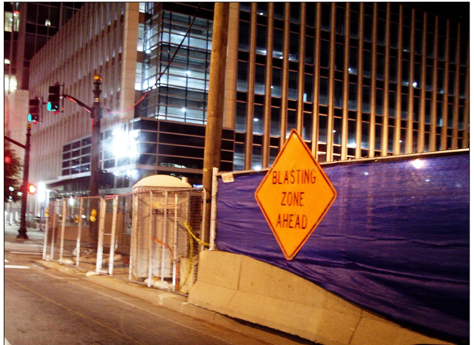
Above: Cleared of spider webs, the future site of The Diner sits with no construction activity. With the infestation cleared, legal issues with the demolition continue.
